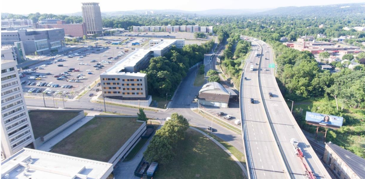
Aerial view at Van Buren St looking south
